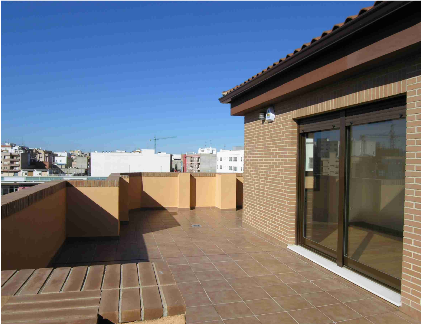
Terrace from Outside Penthouse J
