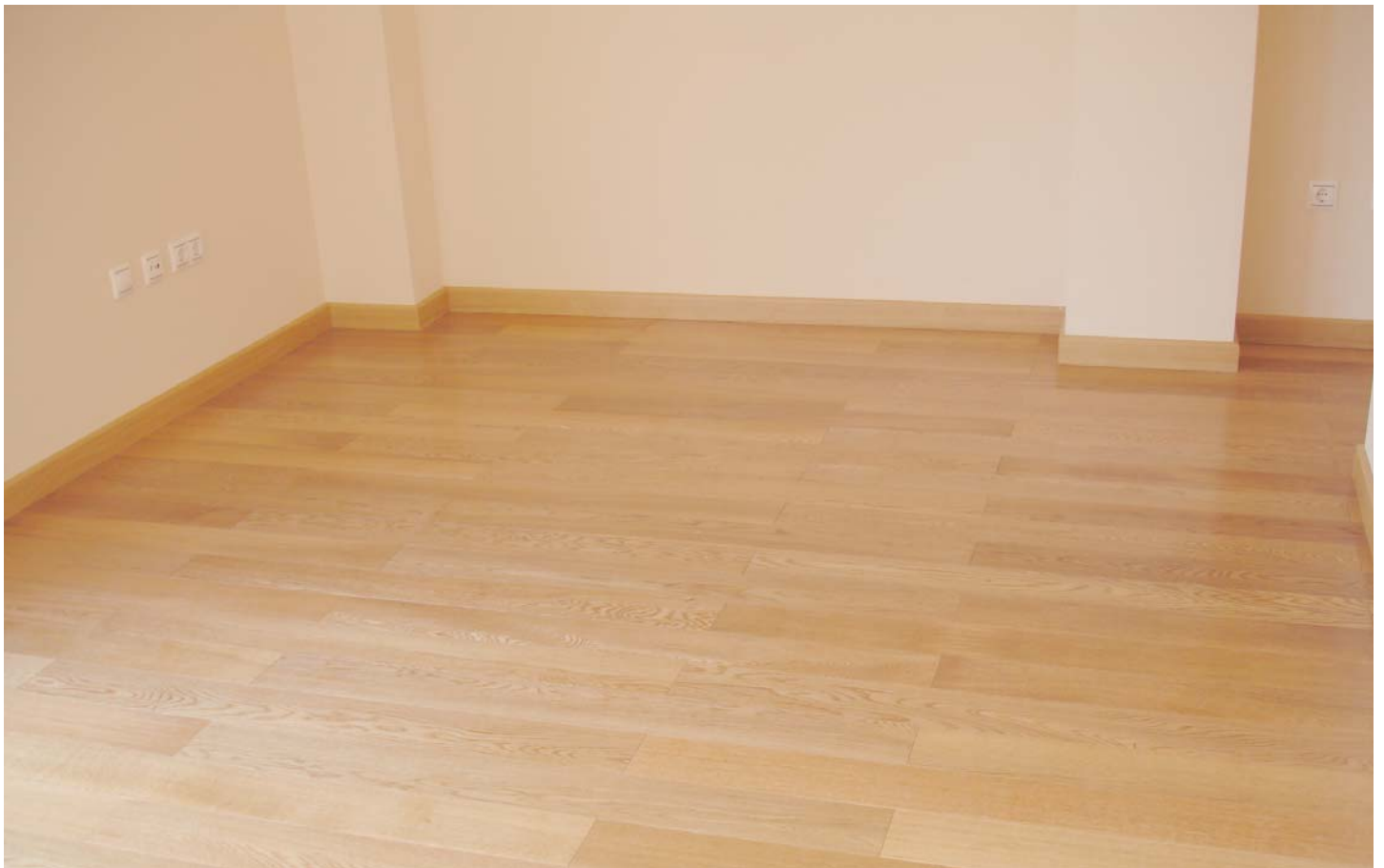
Parquet pavement in top flats
